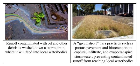
Stormwater runoff is a major source of water pollution in urban communities across the United States. Traditionally, stormwater is drained through engineered collection systems, or "gray infrastructure," and discharged into nearby waterbodies. As stormwater moves through the landscape, it transports trash, bacteria, heavy metals, and other pollutants from the urban environment — contaminants that degrade water quality and threaten public health. Stormwater
